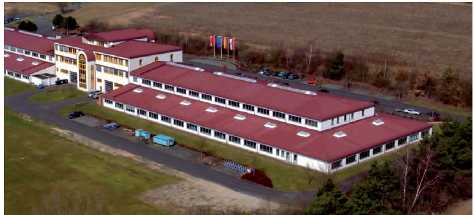
Eichenzell plant (Hesse) with approx. 11,000 m 2 of production, warehousing and office space
