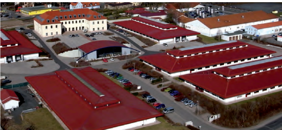
Dermbach plant (Thuringia) with approx. 14,000 m 2 of production, warehousing and office space
